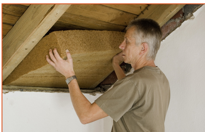
'Vapour open', breathable materials such as natural fibre insulation help to regulate humidity and improve indoor air quality
