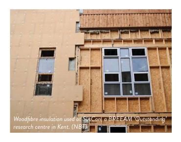
high thermal mass relative to other types of insulation. This is due to the inherent physical properties of the cellulose or protein based fibres and significantly enhanced by the presence of chemically bound water contained in these fibres. Water has a very high heat capacity which is twice that of concrete so its presence in natural fibres adds to the ability of the insulation to absorb heat energy.
