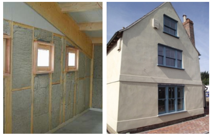
Natural fibre materials are often used in conjunction with mineral products such as lime renders.
